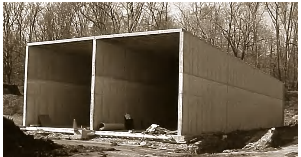
Figure 5. Forced-aeration composting bunkers under construction.
